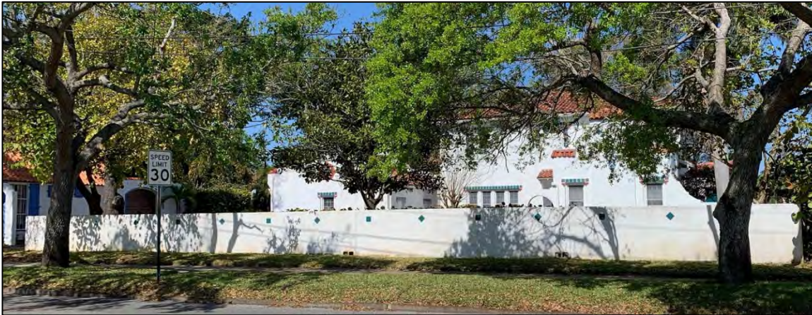
Figure 4: Photograph of the wall along the streetside of 2240 Coffee Pot Blvd NE. Wall is setback 6.5 feet from the sidewalk. Photograph provided by applicant.
