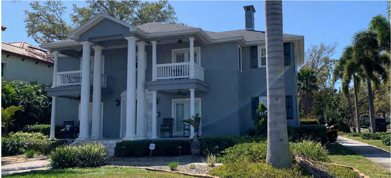
Figure 12a. Property Exhibit D, 2430 Coffee Pot NE: east elevation and front, looking west (from Coffee Pot Blvd NE)
