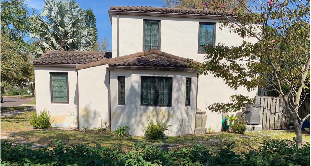
Figure 8. South Elevation-Right Side, 2209 Brevard Rd NE, looking north: new 4' 8" h wall around perimeter, 4' setback from 22 Ave NE sidewalk
