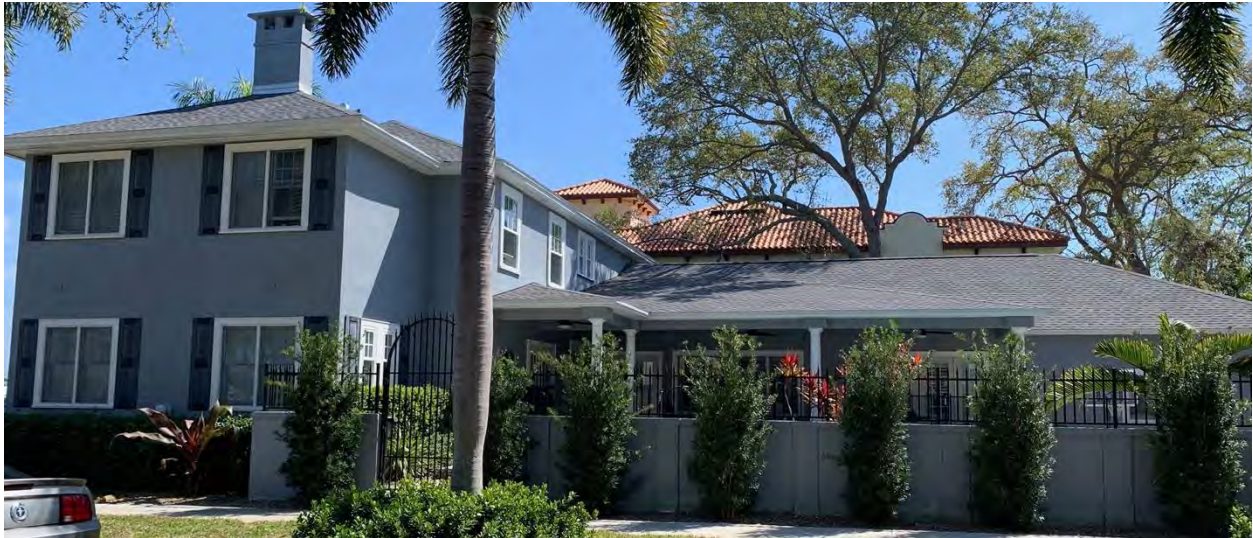
Figure 12b. Property Exhibit D, 2430 Coffee Pot NE: north elevation and right side, looking south (from 25th Ave NE)
