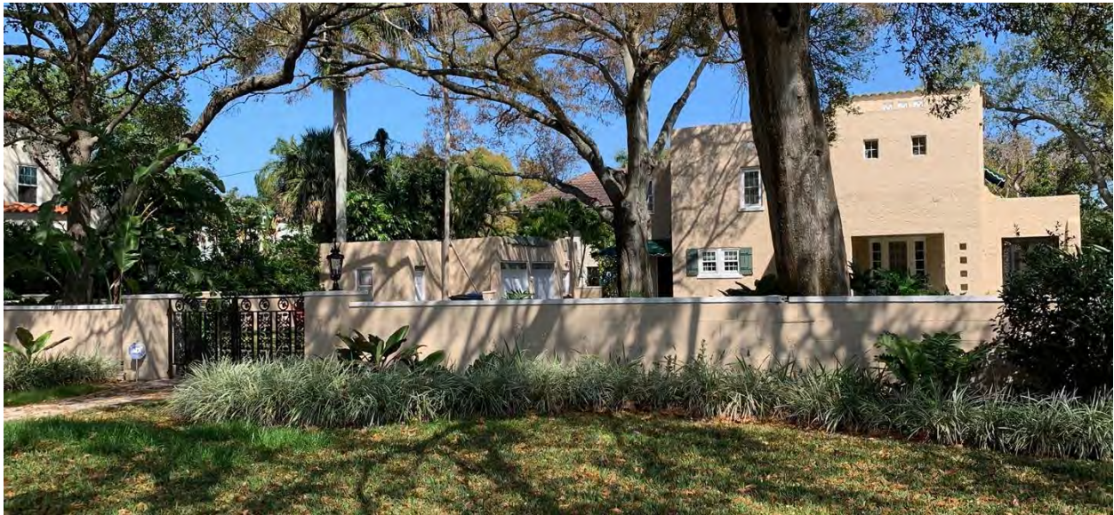
Figure 10b. Property Exhibit B, 215 23rd Ave NE: west elevation and left side, looking east (from Andalusia Way NE)
