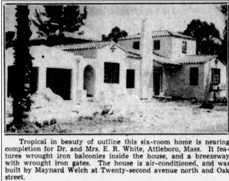
Figure 1: Image of 2209 Brevard Rd NE under construction. From the St. Petersburg Times , April 2, 1939.
